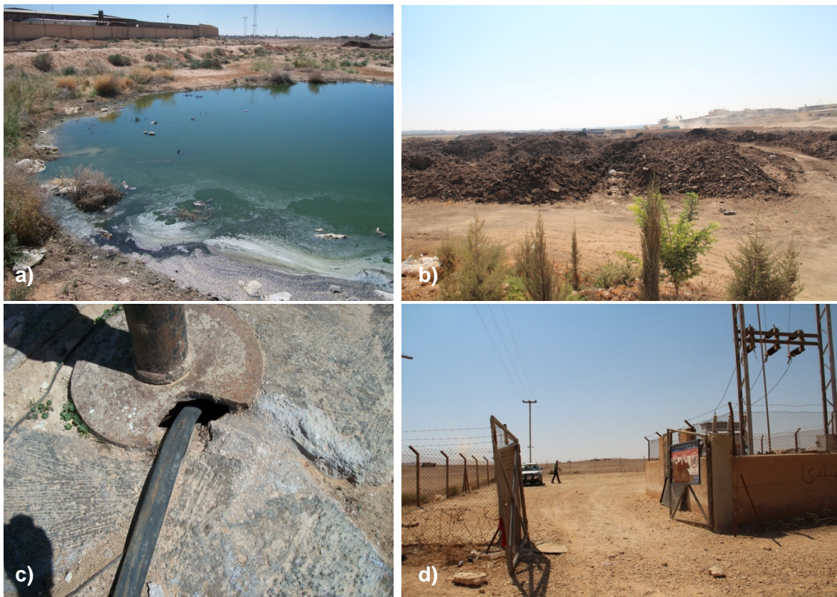
Fig. 66: a) wastewater disposal, b) cow manure dump, c) open borehole allowing direct contamination, d) open/broken fence around groundwater wells with Bedouin camps next to it. (Picture taken around Hallabat wellfield by H. Kirsch, 2012, and A. Steinel, 2011).
