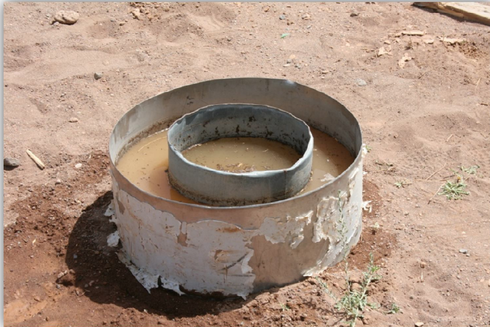
Photos 16, 17: Implementation of third DRIT in Wadi Hassan.
