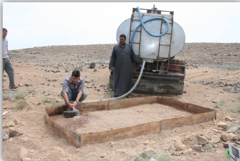
Photos 23, 24: Installation and implementation of BIT in Mafraq Safawi Eastern site.
